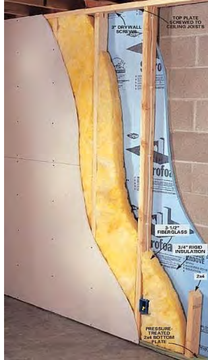
Figure 3-4: Brick Wall with Furring Details
