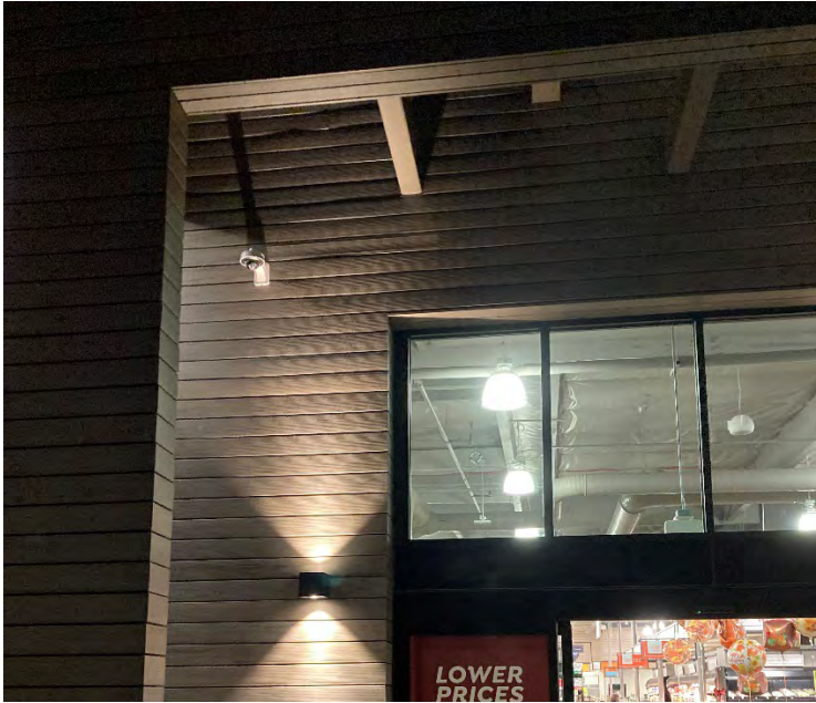
Figure 6-2: Example of a Security Camera That Does Not Qualify for Additional Lighting Power Allowance for Security Cameras
