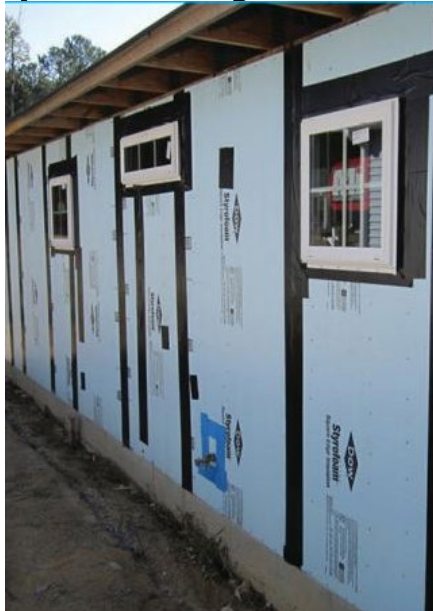
Figure 3-19: Properly Installed Rigid Insulation with Sealant Tape
