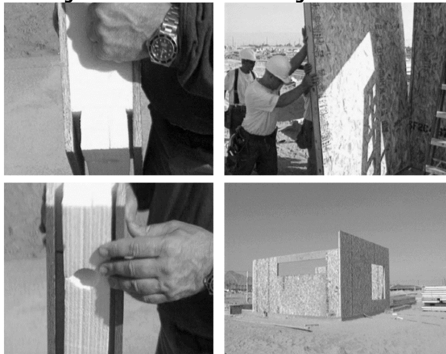
Figure 3-53: Methods of Joining SIPS Panels
