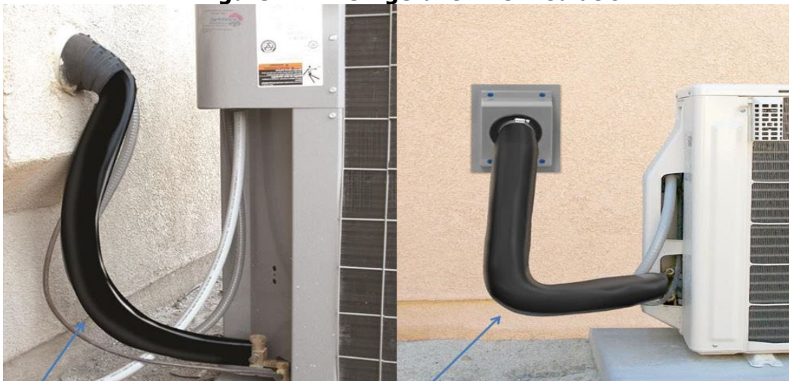
Figure 4-1: Refrigerant Line Insulation
