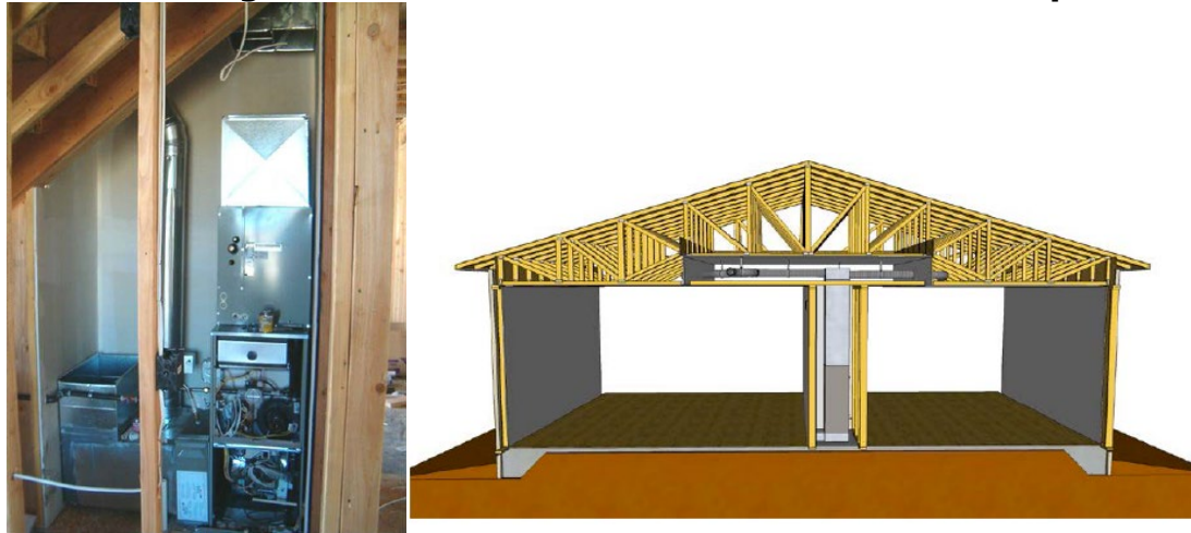
Figure 4-14: Mechanical Closet Placement Example
